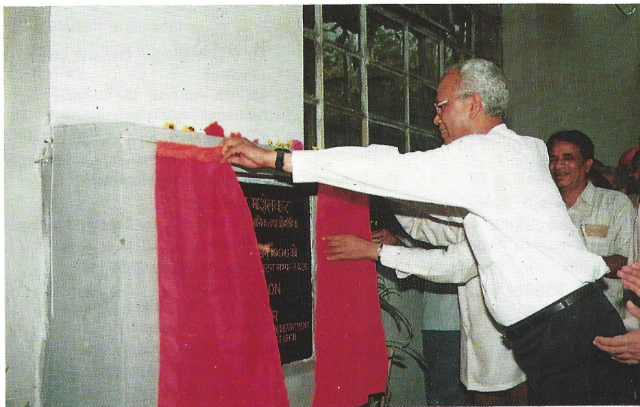
Dr R A Mashelkar, DG SIR, inaugurating the 33 KV sub-station at IIP during his visit.
